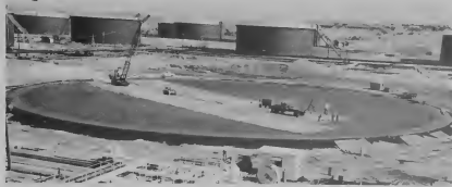
THIS FOUNDATION of a huge crude tank with other tanks in background may give an idea of its size.
